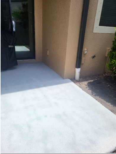
Photo 1: Photo showing downspout from roof gutters recently installed.
